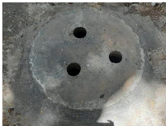
Figure 4-3: Percolation pit for ground water recharge
