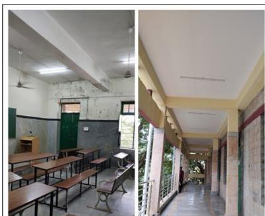
Figure 5-4: LED lamps used in the class rooms
